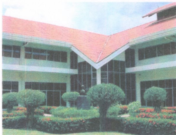
BUILDING COURT YARD (O.P.D.)
